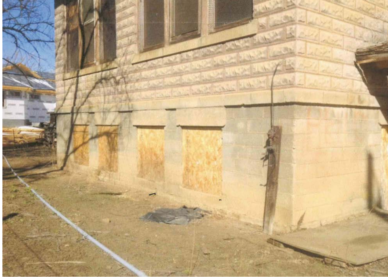
EXISTING SIDE | REGRADING FOR DRAINAGE, APPROX. 10" ABOVE EXISTIN GRADE. WINDOW WELLS TO BE ADDED, SEE PAGE 8 [ALL SIDES]
