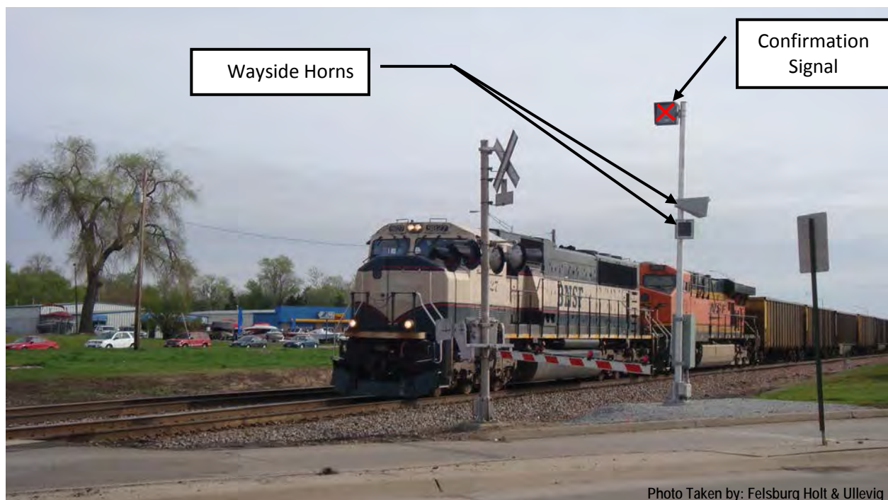
Figure 10. Highway-Rail Crossing Equipped with Wayside Horns
