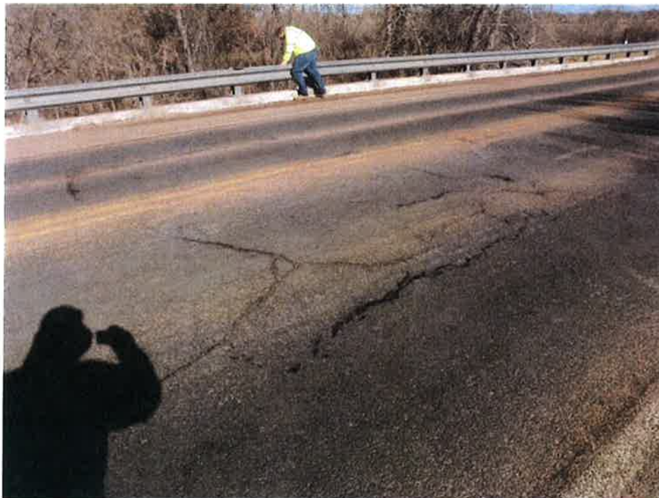
LIGHT ASPHALT CRACKING ON DECK
