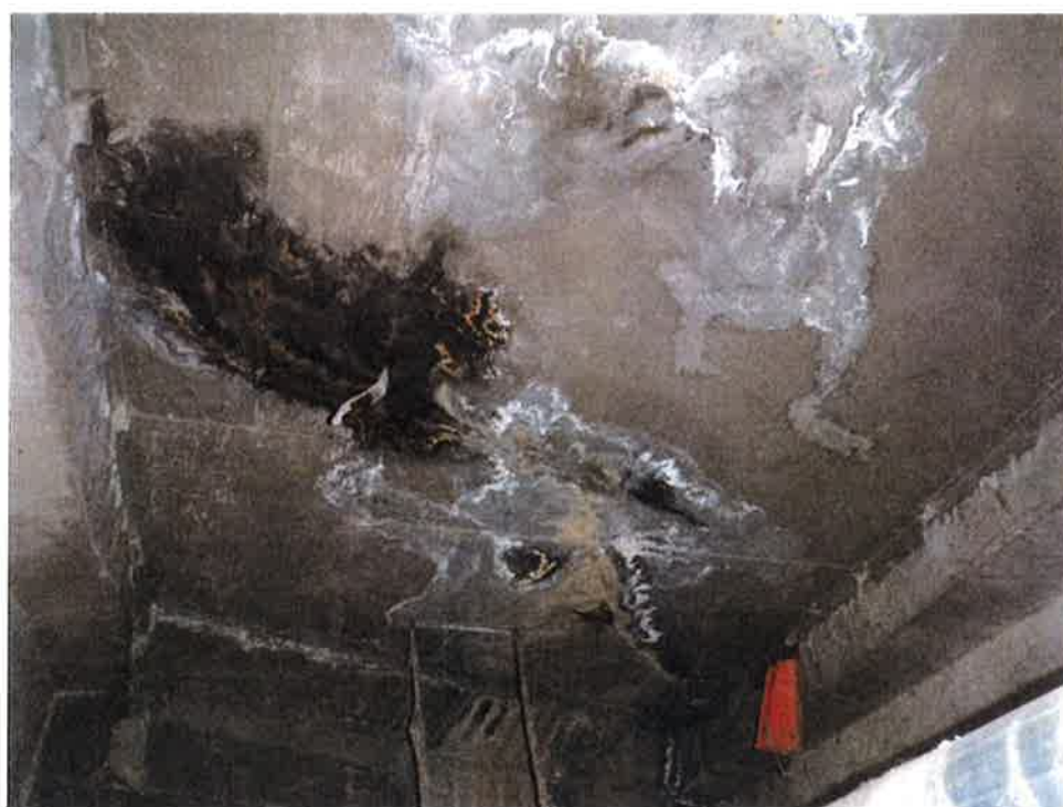
TYPICAL CRACKING WITH LIGHT EFFLORESCENCE AND RUST STAIN IN SOFFIT
