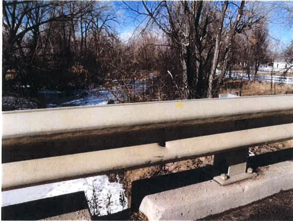
SMALL HOLE ON WEST SIDE OF FLEX BEAM
