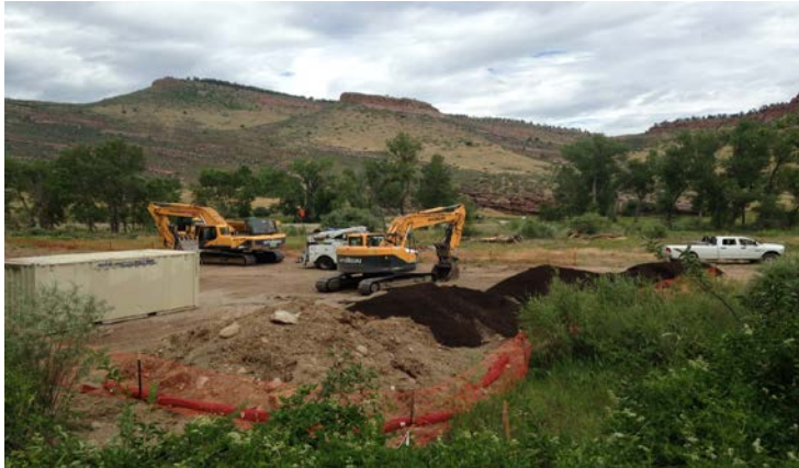
Main staging area
