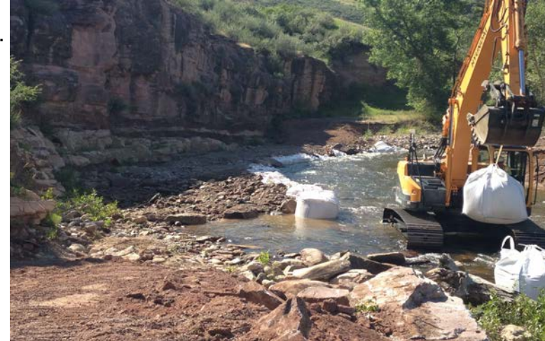
Construction of Temporary Low Water Crossing to material disposal site.
