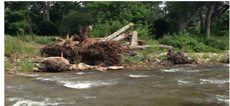
Woody material staged in preparation for large woody structure installation at main channel St. 56+50
