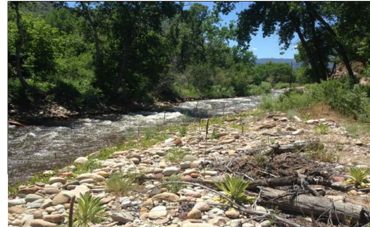
Before Construction: Confluence of main channel and overflow channel F looking upstream
