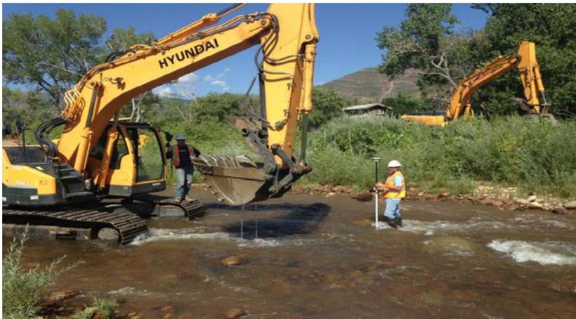
Setting elevation of riffle crest St. 65+09
