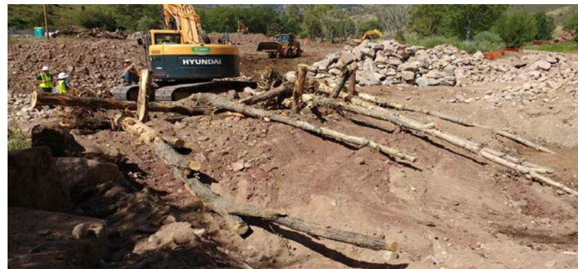
Installation of Type 5 Large woody structure at 70+50
