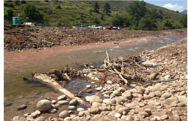
Upstream view: Installation of Type 1 Large woody structure at 71+90
