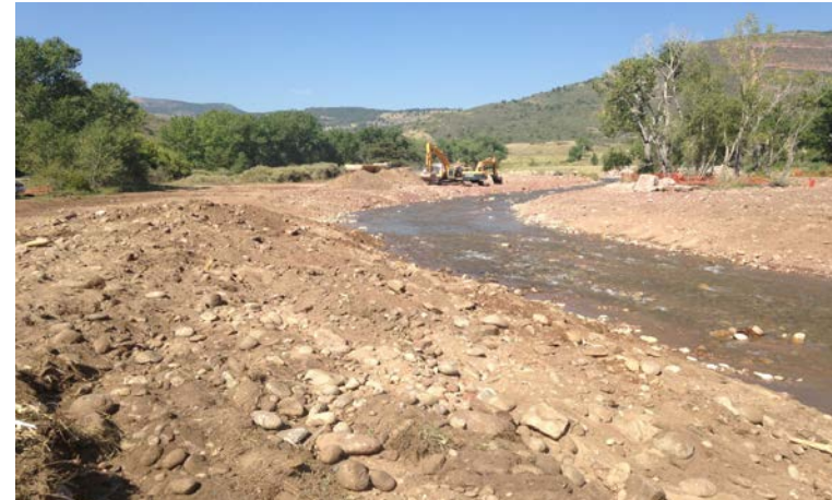
Downstream View: Floodplain benching adjacent to main channel St. 66+50 to 77+00.
