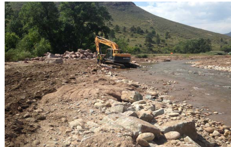
Upstream View: Boulder toe bank stabilization between main channel St. 66+00 to 70+80
