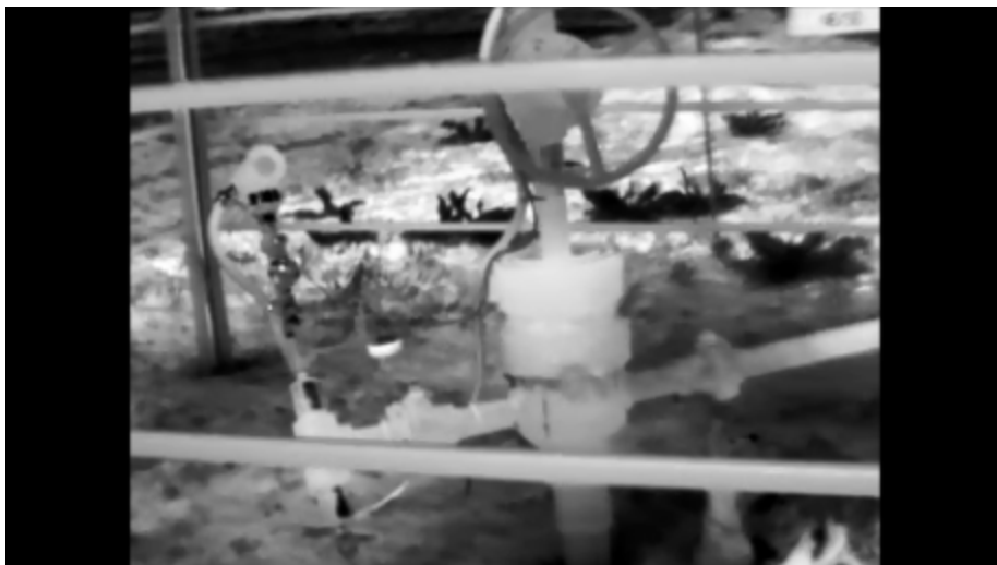
Figure D5. Emissions from tubing hanger on wellhead
