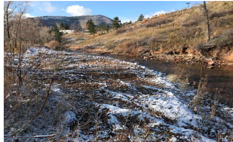
Upstream View: Right floodplain grading adjacent to main channel St. 33+80 to 35+50.
