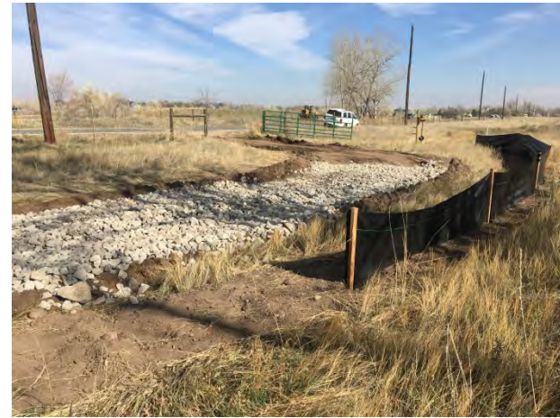
11-03-17: Installation of rock for Gage access road improvement and VTC installation
