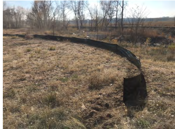
10-27-17 Silt fence installed at Gage property (Hygiene Rd Access to South)
