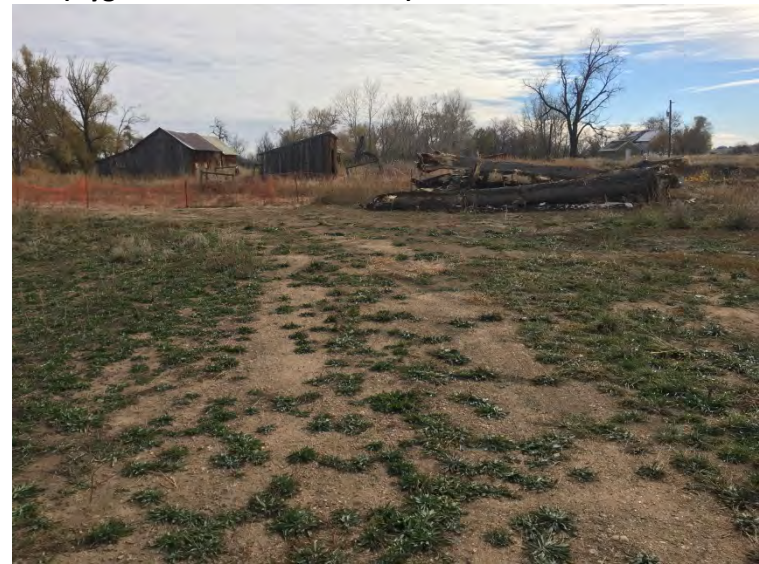
10-27-17 Construction perimeter fencing and first wood delivery at Ramey access point near 61st
