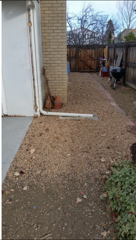
South side yard and chimney above helical piers.
