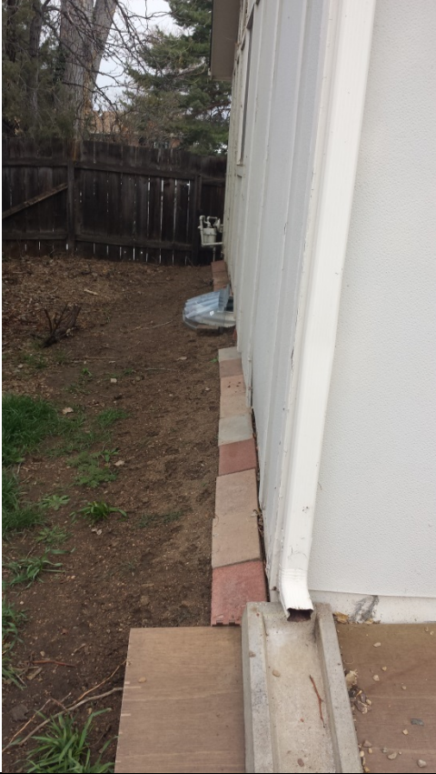
Temporary grading measures.
