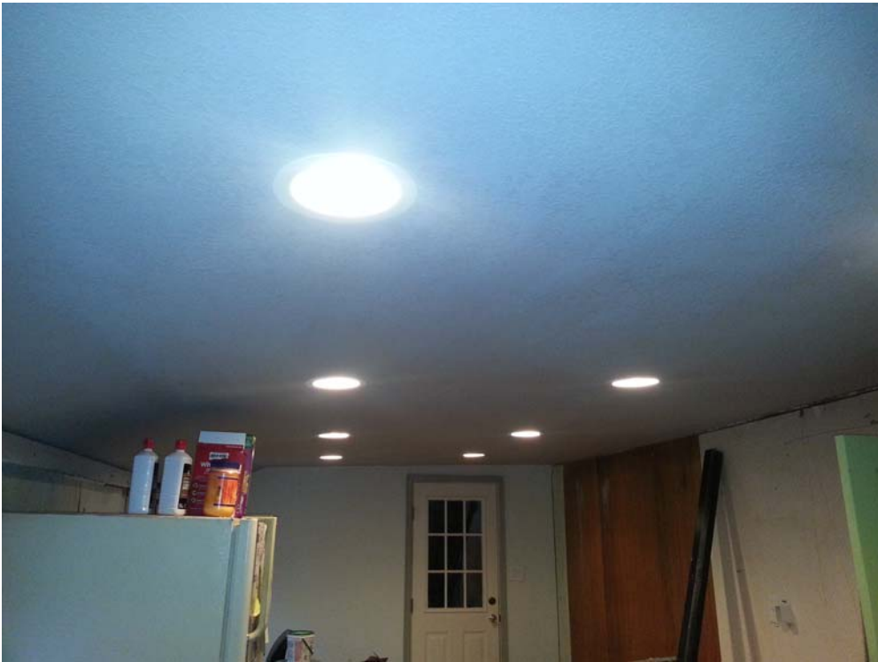
Ceiling in kitchen
