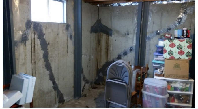
Completed structural bracing and epoxy repair at basement walls.
