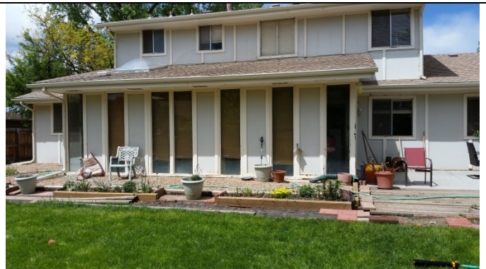
Back elevation with new concrete patio, drainage. And gutters.
