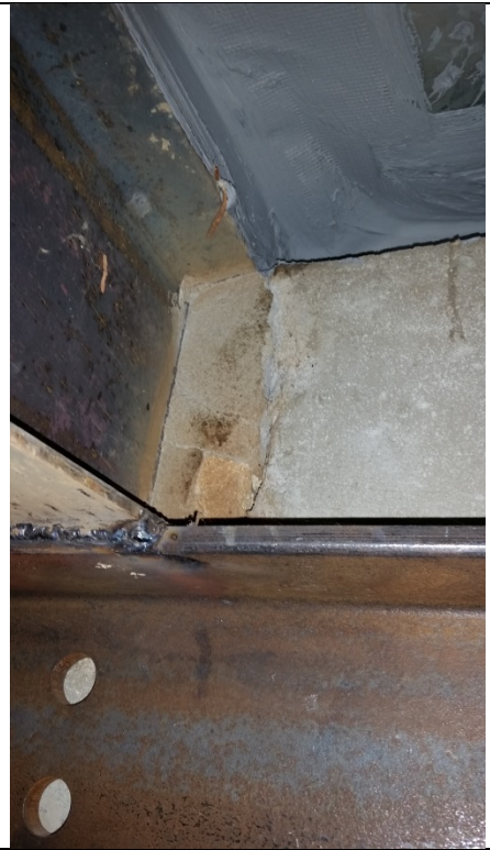
Structural brace for existing steel beam.
