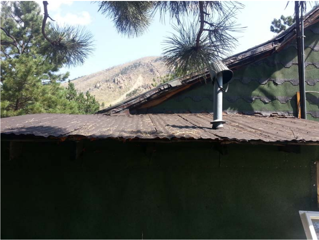
Roof over bathroom
