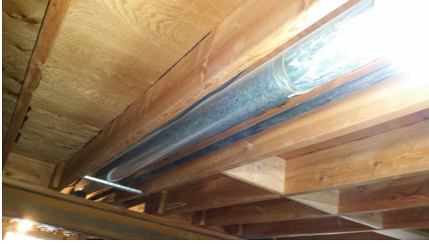
New blocking at basement.
