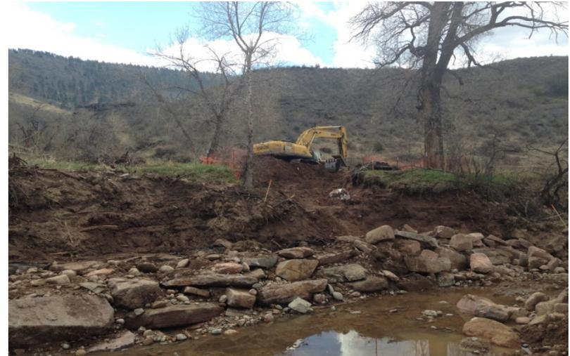
**Looking upstream: Excavation of low water crossing ditch outfall tie-ins in progress.**
