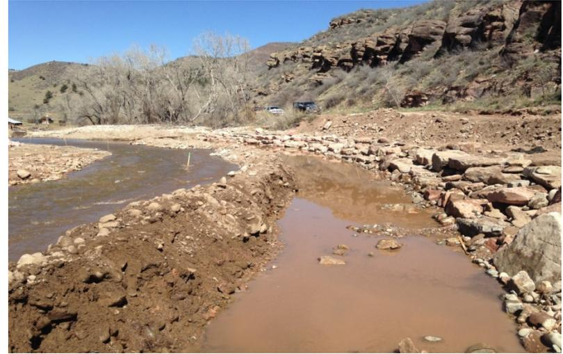
**Looking Downstream: Completed construction of boulder toe bank stabilization .**
