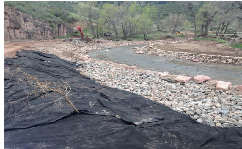
**Looking Upstream: Installation of 9 inch rip rap behind boulder toe and above separation geotextile.**
