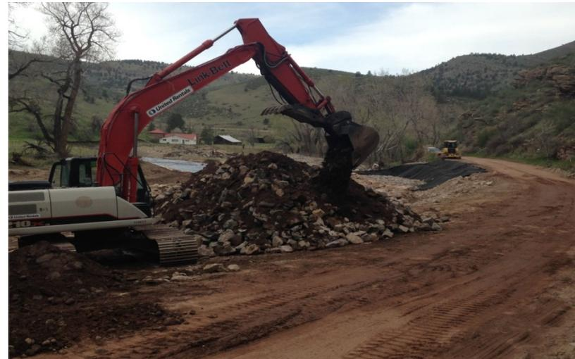
**Batching Soil riprap mix (65-35) for bank stabilization.**
