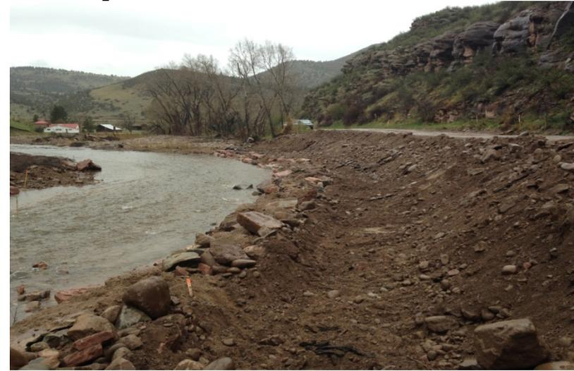
**Looking Downstream: subgrade preparation for bankline construction.**
