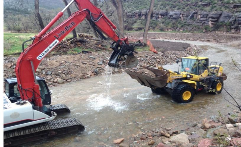
**Looking downstream: Completing construction of low flow channel and hauling excess material for processing.**
