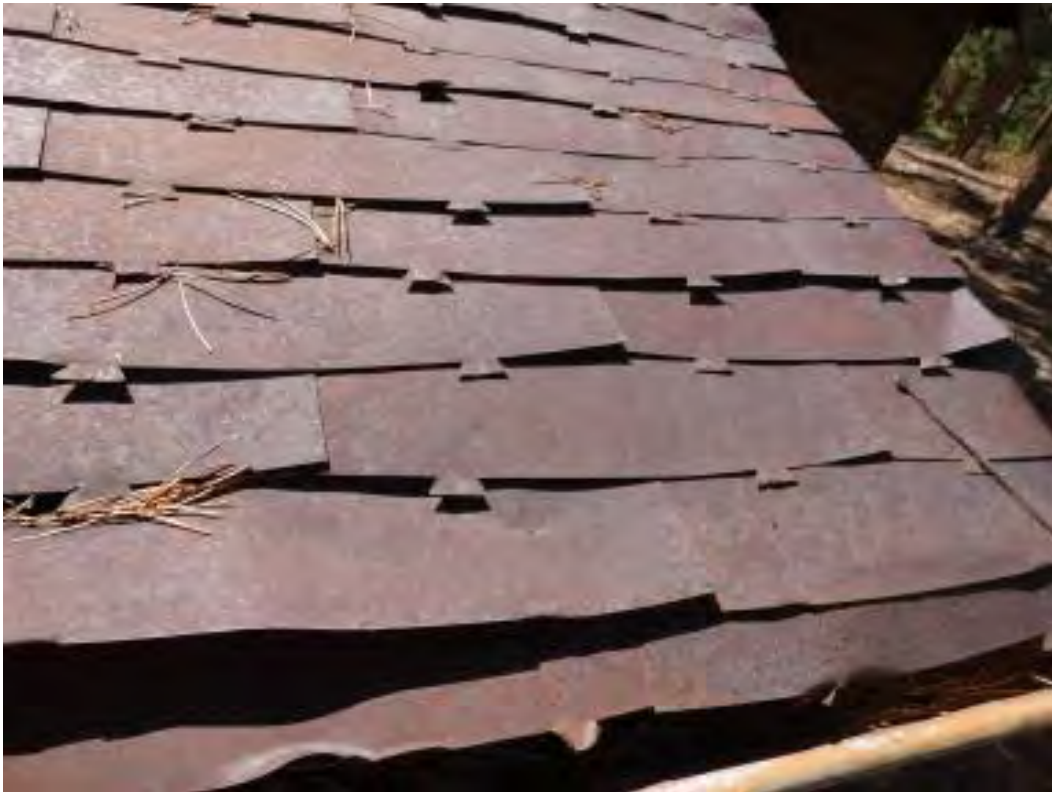
Detail view of metal shingle roofing seen on garage, privy, and shed
