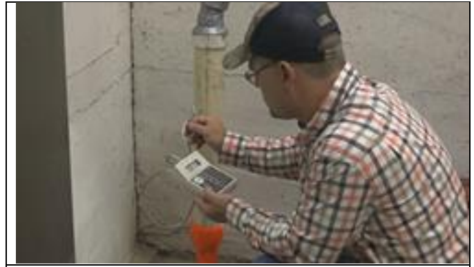
Air Flow Measured to Determine Fan and Vent Pipe Size
